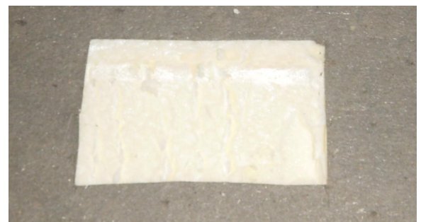
Figure 4 - Cut out insulation facing
