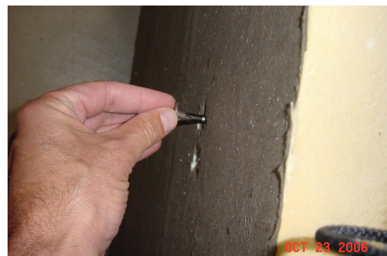
Figure 8 - Installing T-Nut
